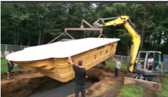
OPTION 1: MECHANICAL EXCAVATOR (8T excavator)
