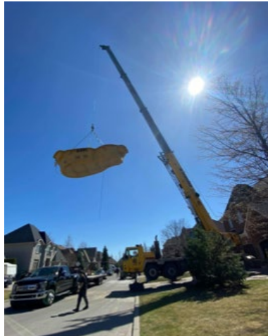
OPTION 2: Crane (45tons) (Pool weight 1500LB)
