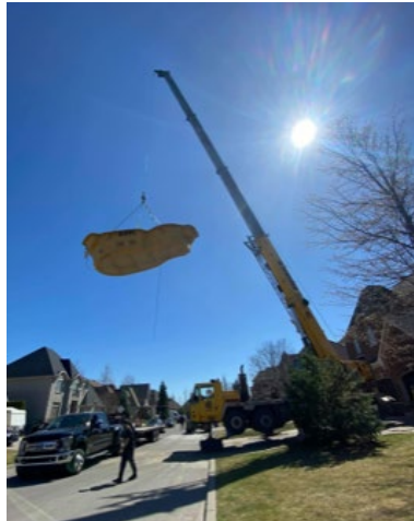
OPTION 2: Crane (45tons) (Pool weight 2800LB)
