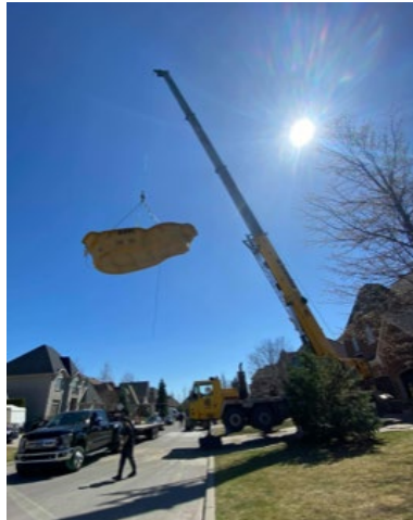
OPTION 2: Crane (45tons) (Pool weight 2800LB)
