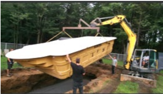
OPTION 1: MECHANICAL EXCAVATOR (12T excavator)
